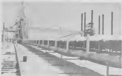
The 660-ft. yard belt of sulfur stacker. Fahá di 660 pia largo pa transporta azufre.
